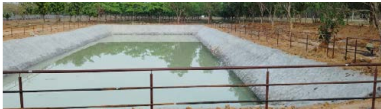
Rainwater collection pond constructed to reuse water into domestic purpose.
